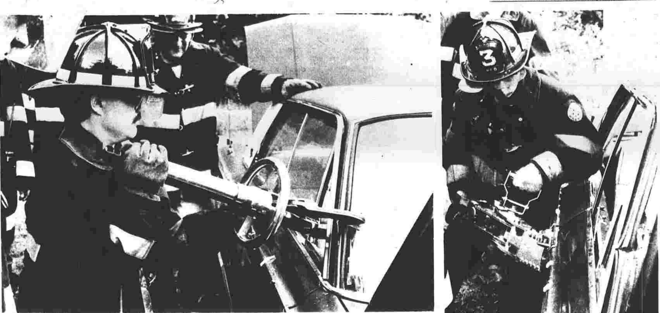
Garry Albert, left, a firefighter with the Eighth District Fire Department, Monday demonstrates the use of shears that are a part of a new tool the department has acquired for rescuing victims trapped in automobiles. The shears are used to cut off the post at the windshield so that the roof can be rolled back. At right, Don Moore, another volunteer firefighter, uses a spreader tool that comes with the extrication package to pry open the passenger door of the car. The Gator Tool package has been purchased by the district for $5,200 to supplement the Hurst tool now in use. According to Thomas O'Marra, spokesman for the department, the hydraulic tool is powered by its own air supply and operates quietly, permitting medical personnel to communicate with a trapped victim. O'Marra describes the new tool as a light-duty extrication tool. It applies 12,000 pounds of pressure at the tip of the spreader.
